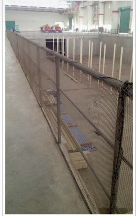
NET FOR HANDRAIL MACHINE PIT
